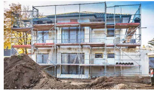
SMALL BUILDING SITES
